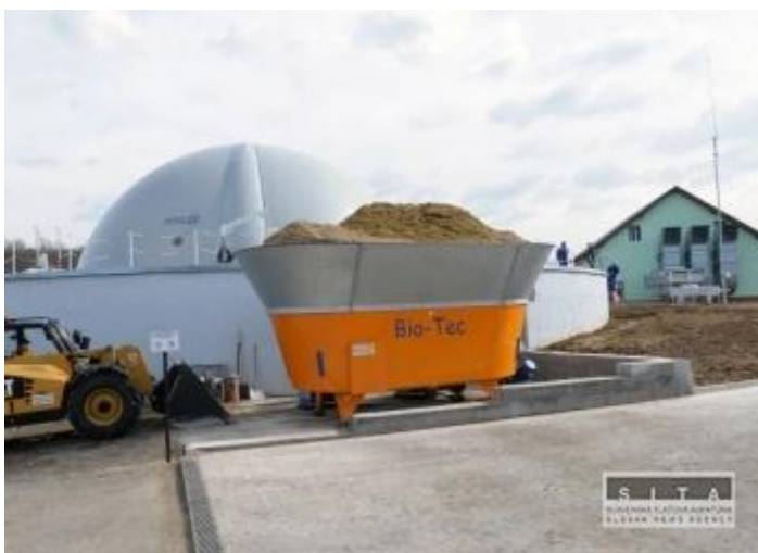
Figure 23.8. Biogas station in Rozhanovce (East Slovakia)
